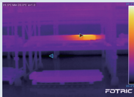
Battery Energy Storage System (BESS) Thermal Runaway Early Warning
